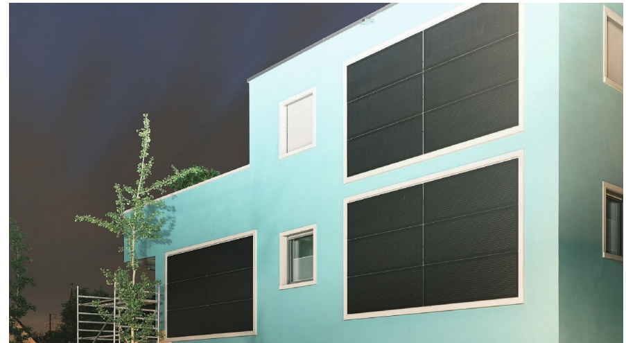
Photo: Unterwerk Stenna (top); MFH Nordtorweg (bottom). Credits: Yufei He / BUK ETHZ
