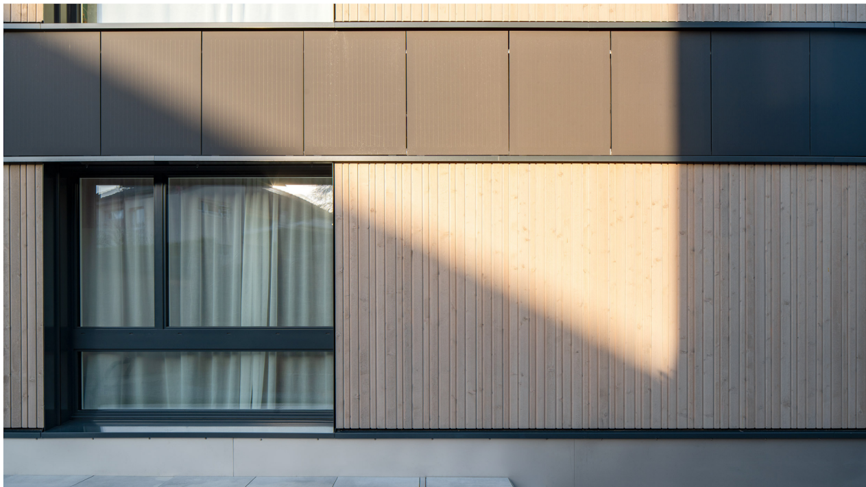
Building front. The matt-brown photovoltaic modules matches nicely the wood cladding.
