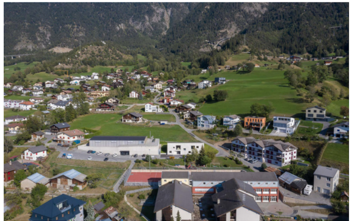
The building functions as a pivot, resolving both the street corner and the direct relationship with the sports centre.
