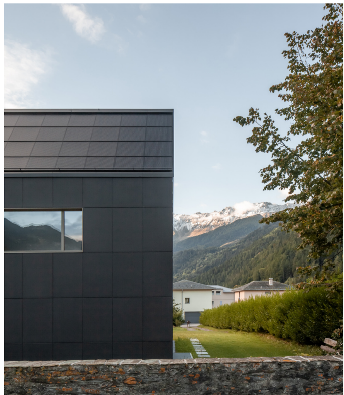
The complete building envelope consists of integrated photovoltaic modules.
