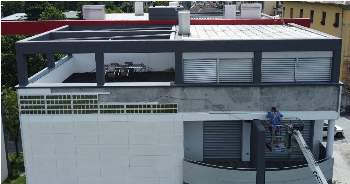
Figure 3 Installation of Horizontal H profiles
