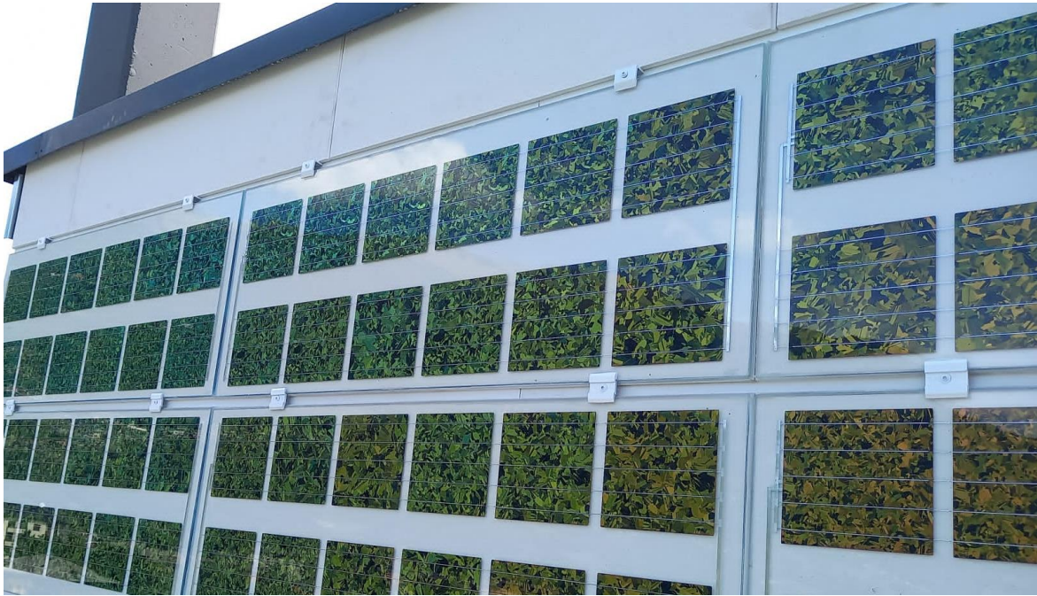
Figure 4 Aluminum safety clamps installed to provide extra safety
