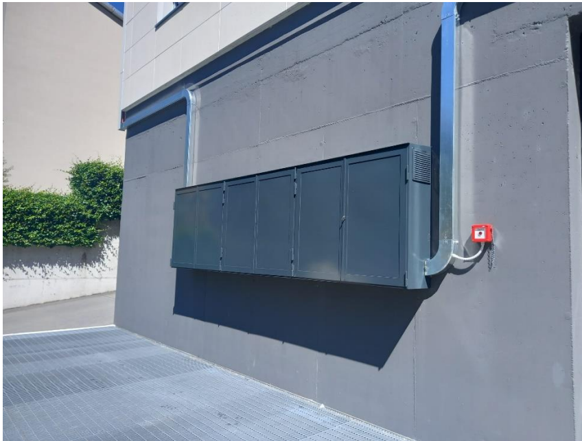
Figure 9 Steel cabinet for electrical equipment
