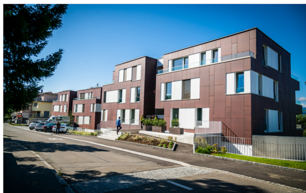
The two new buildings as seen from the street. The facade cladding consists of red and white photovoltaic modules.
