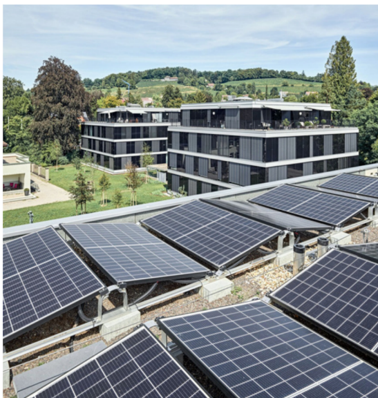
View of the roof with the photovoltaic installation.
