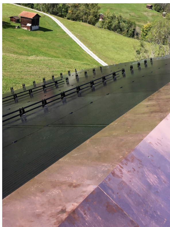
The roof is detailed with copper elements. Photo source: Solpic AG.
