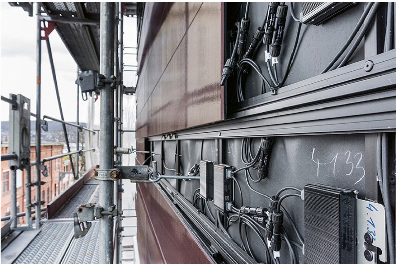
Installation of photovoltaic modules.
