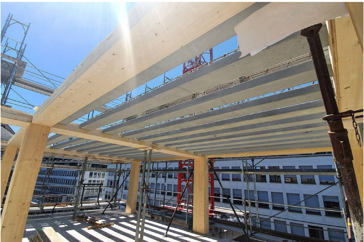
One of the special features of the building is the skeleton construction in wood-concrete hybrid technology. Photo credits: Häring AG.
