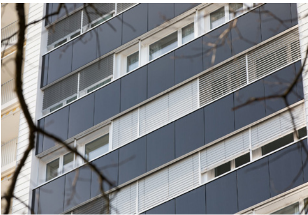
Black photovoltaics modules are ideal for a simple and understated facade design
