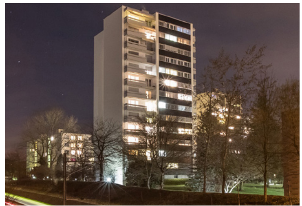
The photovoltaic modules blend in smoothly with the basic architecture of the building.
