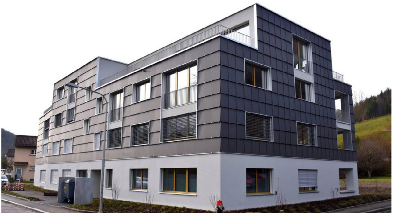
The facade is almost completely covered with solar modules. Photo: Pascal Wiederkehr.
