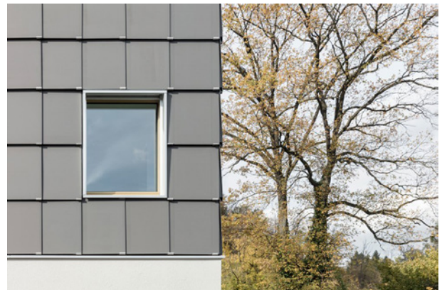
The cell structure disappears behind the light printing on the matt front glass. Photo: Pascal Widerkehr
