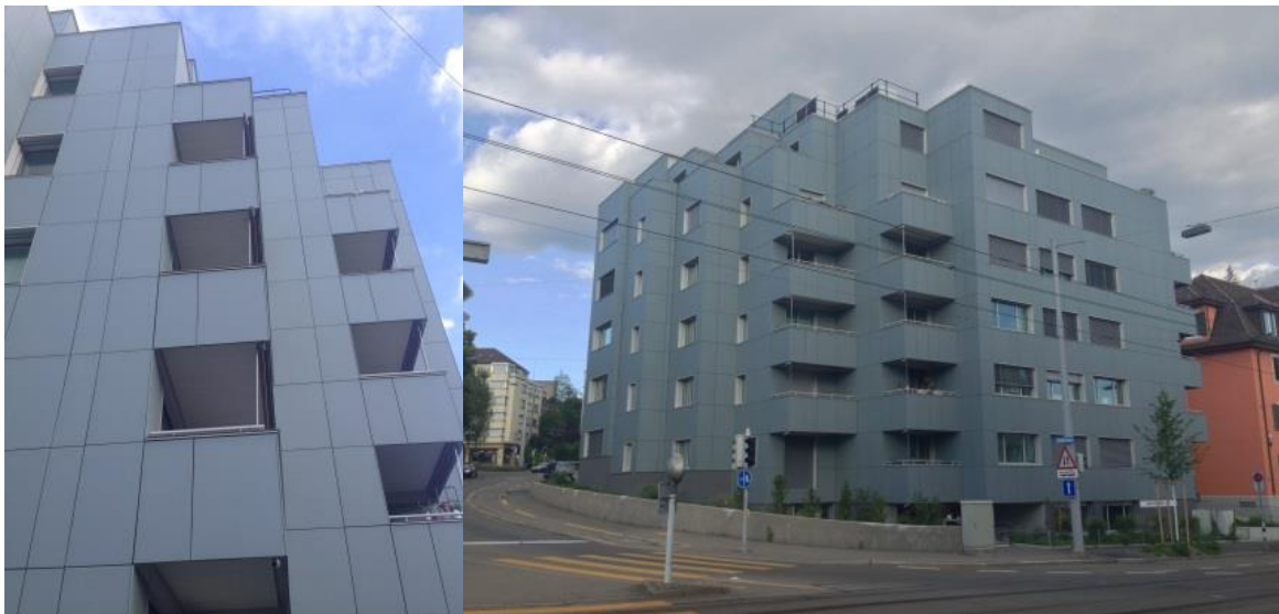
Figure 29: Project Pilot Plus-Energy Building Renovation – Zürich. Coloured frameless BIPV glass modules treated to obtain an anti-reflective and matt surface have been used to cover the whole building envelope [30] (Source: Viridén + Partner AG).
