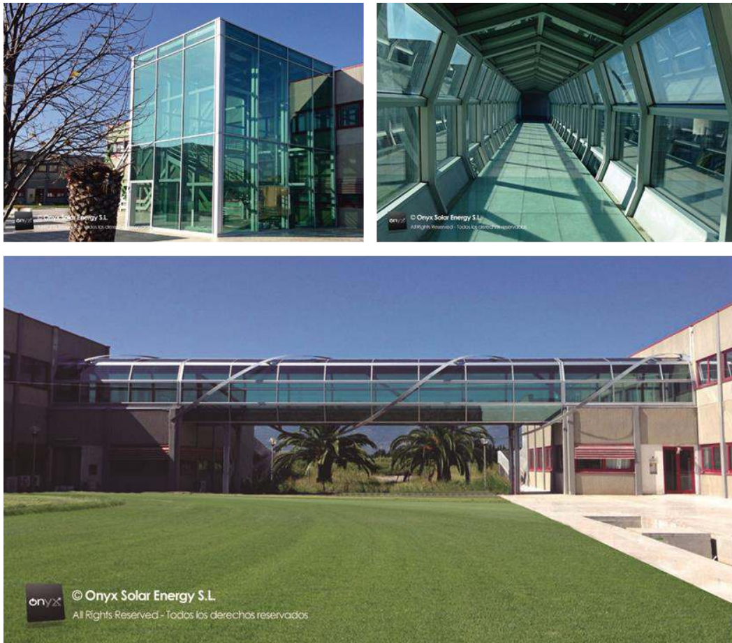
Figure 11: Semi-transparent coloured amorphous silicon BIPV modules used in the refurbishment of the buildings of the Terina Mediterranean Foundation in Calabria (Italy). (Source: www.onyxsolar.com/mediterranean-foundation-terina ).
