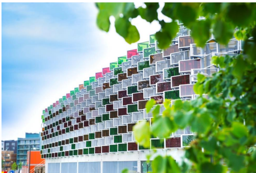
Figure 22: Façade elements with coloured encapsulants using a CdTe active layer (Source: www.soltechenergy.com ).
