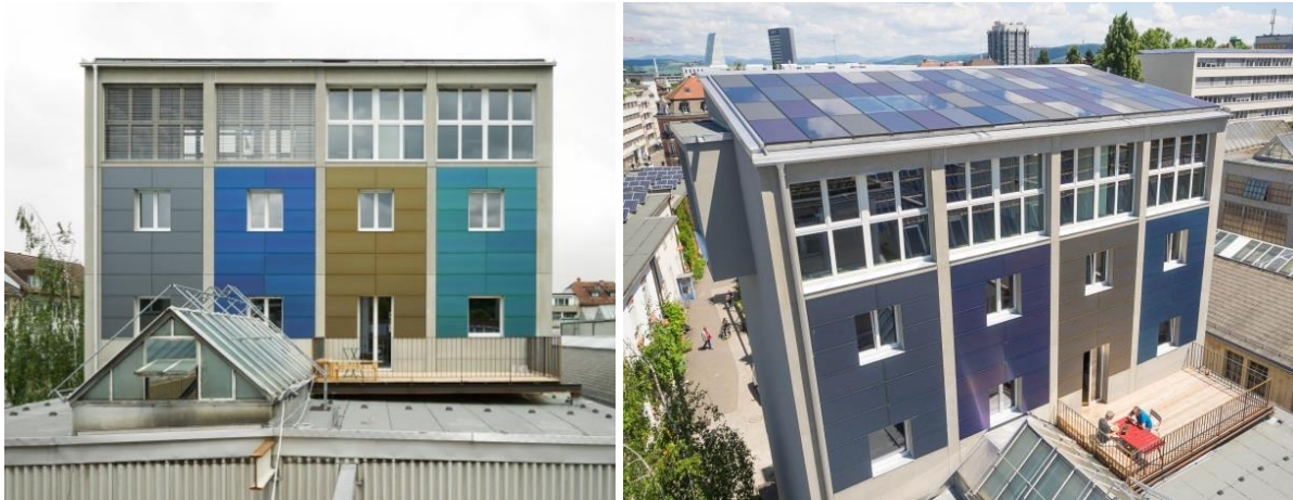
Figure 24: Colourful printed custom-size solar panels for façades applying SwissINSO Kromatix™. Demonstration BIPV projects: a) Solar Silo “Kohlesilo”, Basel (CH). Industrial building placed in the cultural Gundeldingen area; awarded the Swiss Solar Prize in 2015. (Source: SUPSI; http://www.bipv.ch )
