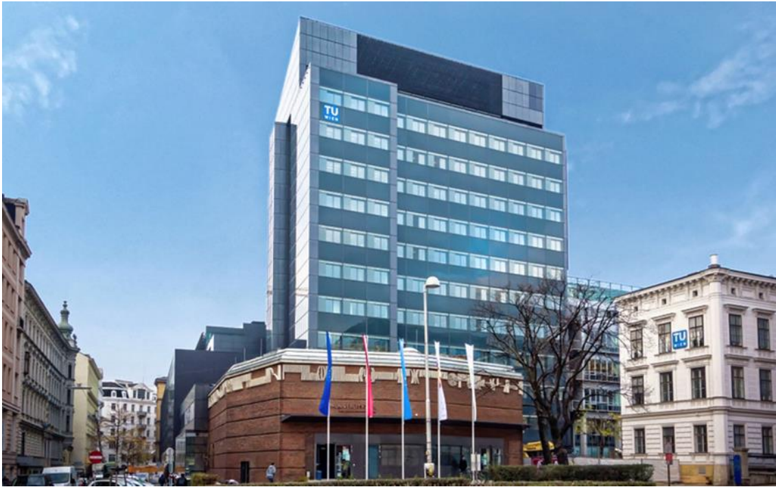
Figure 7: Technical University of Vienna, public high-rise building with BIPV façade; Plus-energy building (Photo ©Schöberl & Pöll GmbH, www.schoeberlpoell.at/en/projects/plus-energy-buildings ).
