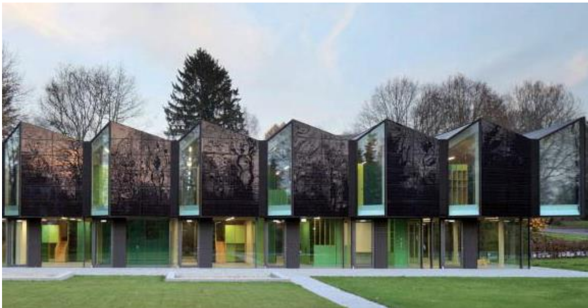
Figure 6: Black BIPV façade with laminated glass on a public building (children’s day-care centre in Marburg); project realized by ertex-solar ( www.ertex-solar.at/produkte/referenzen ) Opus Architekten © Eibe Sönnecken
