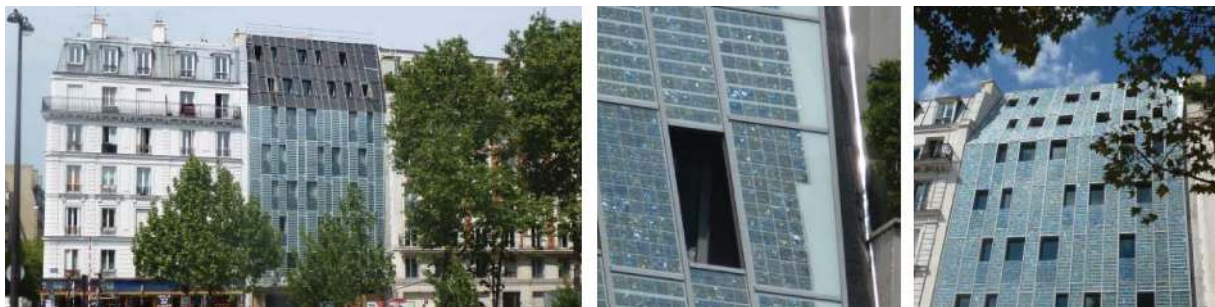
Figure 10: Building with BIPV façade with coloured c-Si cells (LOF), project Fondation Abbé Pierre in Paris ( www.ertex-solar.at/produkte/referenzen );©ertex-solar
