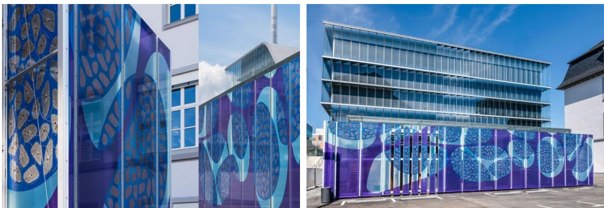
Figure 17: Energy-efficient ETFE-based membrane façade installed using printed Organic Photovoltaic OPVIUS Energizing Surfaces. Source: OPVIUS GmbH and Taiyo Europe GmbH. Press release 29 May 2018, Images: Merck KGaA.
