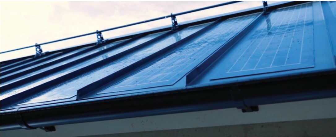
Fig. 2 Detail of the BIPV roof. Source: Midsummer.
