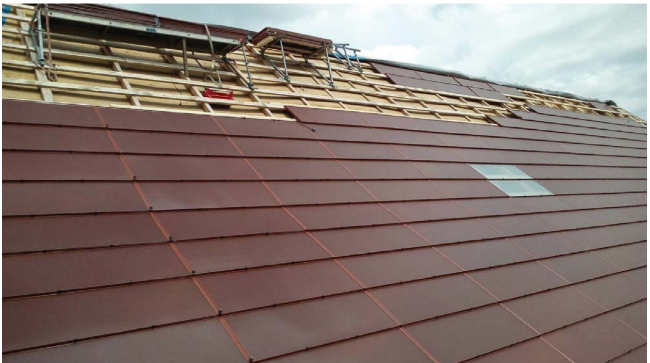
Installation of the photovoltaic tiles. Source: Solstis SA.
