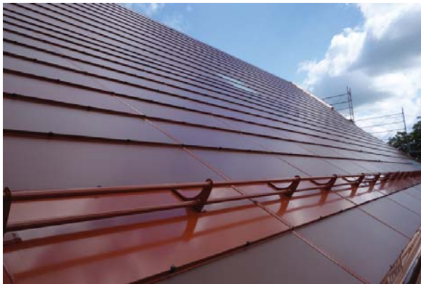
27.2 kWp PV installation made of clay coloured modules. Source: Solstis SA..
