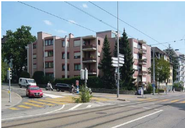
View of the building before the retrofit.
