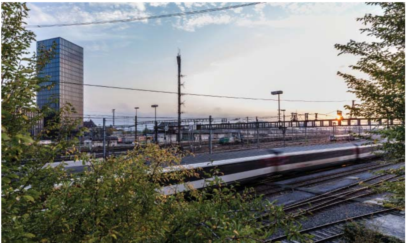
The building is close to the main transport axes.
