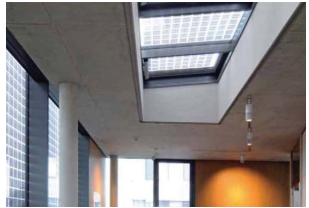
Semi-transparent photovoltaic modules were used on the south facade and on the skylight above the stairwell. Credits: Ertex Solar.
