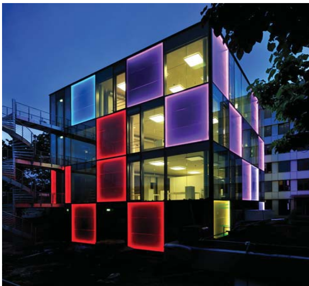
Night view of the building, alongside the transparent PV modules there are also opaque surfaces that can be illuminated at will using different colored-LEDs.
