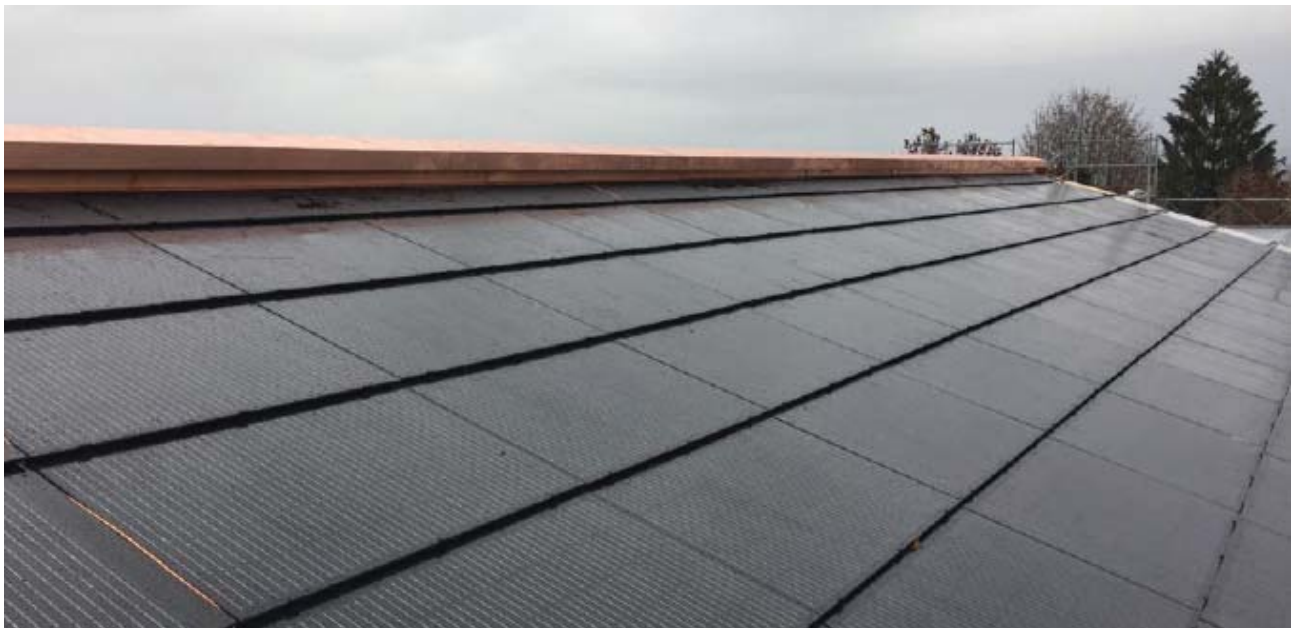
PVT-roof under construction.
