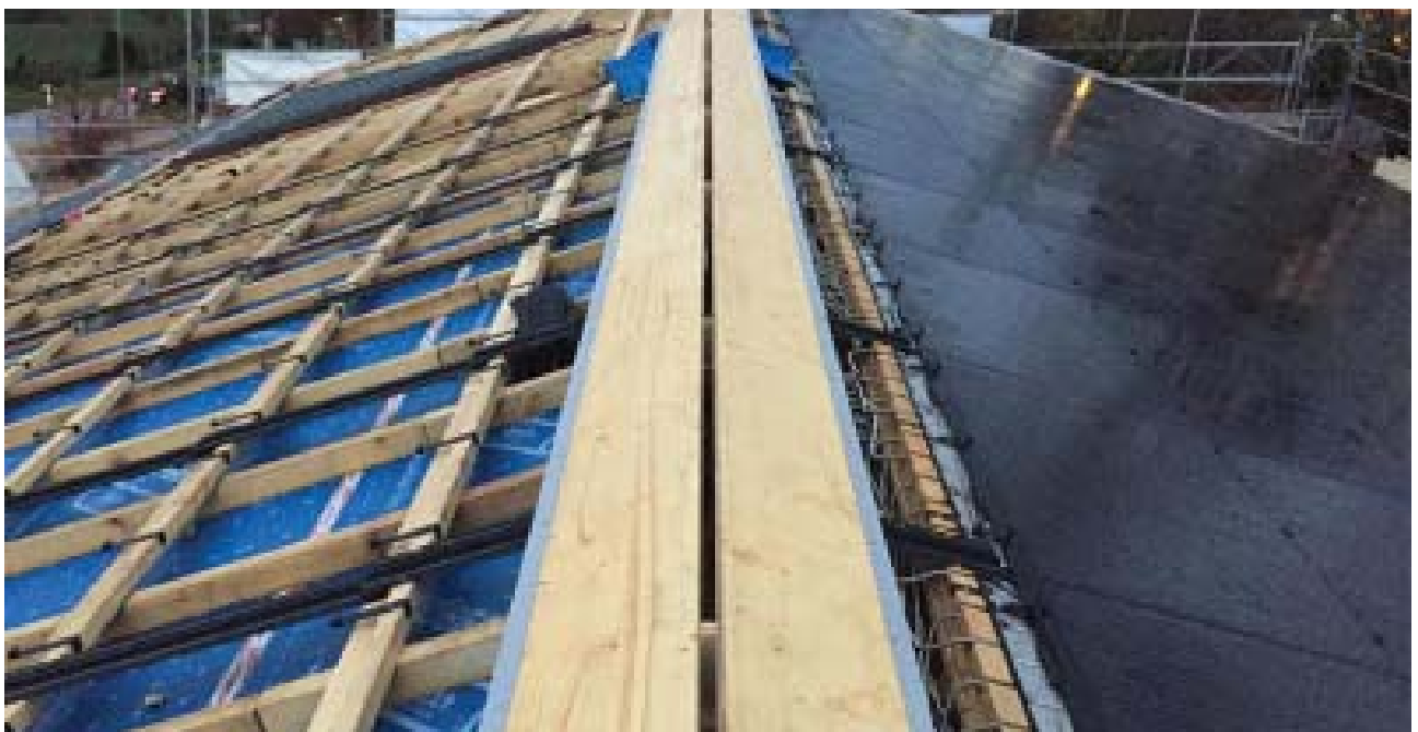
PV-roof (left) and PVT-roof (right) under construction.
