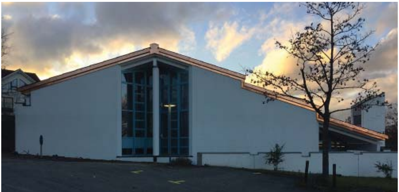
The original edge of the roof had to be redesigned due to the insulation-related increase of the roof area.
