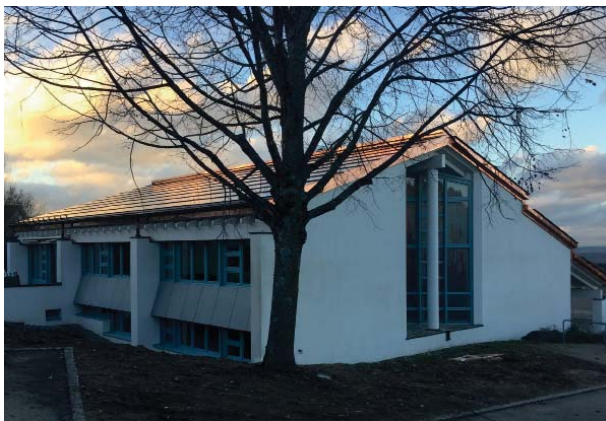
South-east view with PVT roof.
