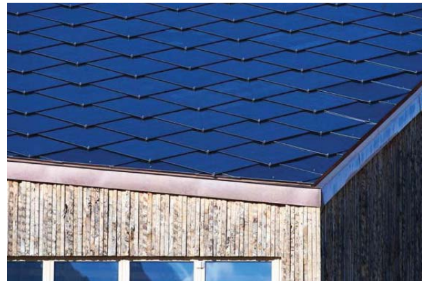
The roof is covered with photovoltaic shingles.
