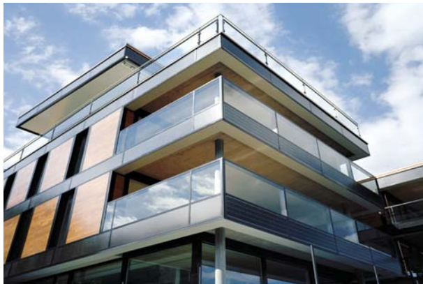
The photovoltaic covered floor courses mark off the horizontal divisions of the elevations.
