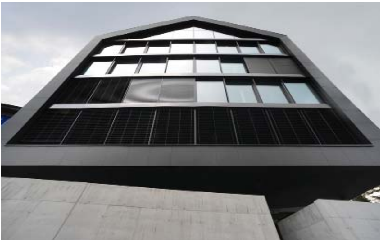
It is practically impossible to distinguish the active PV elements from the facade cladding.
