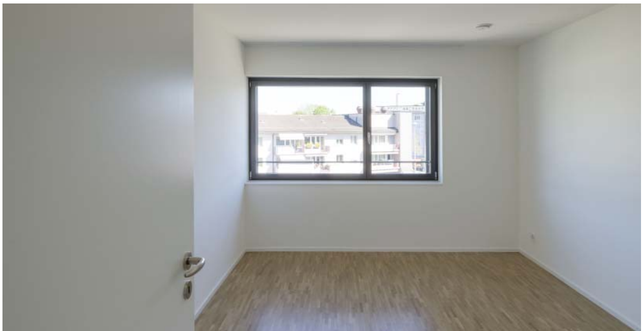
The existing windows have been all replaced.
