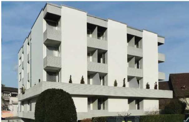
View of the building before the retrofit.
